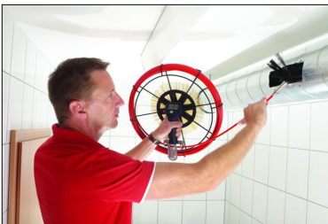
Fig. 21: Cleaning a ventilation duct
